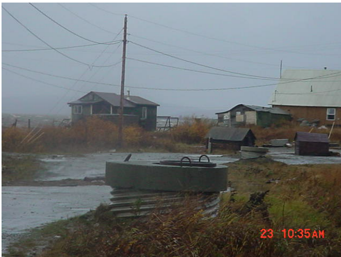
Photo 3: Wind driven waves causing flooding and erosion in Koyuk, Sept. 2005.
